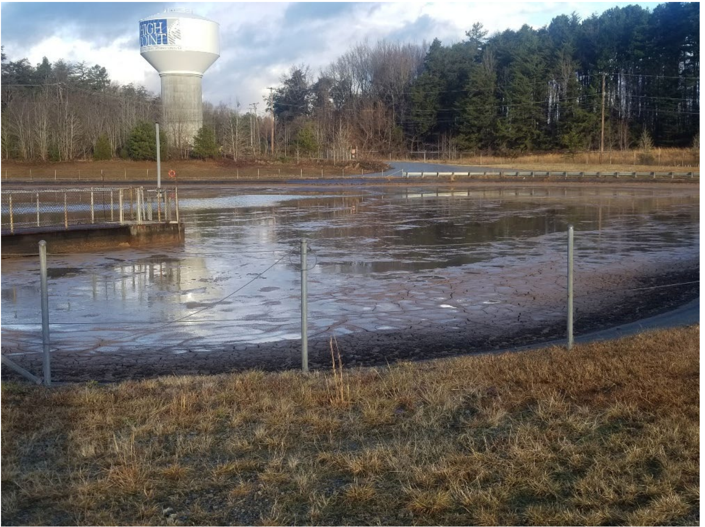
North Lagoon- Ward Water Plant
