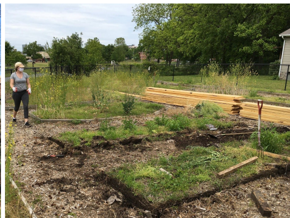
Preparation for new raised beds at Southside Community Garden in May.
