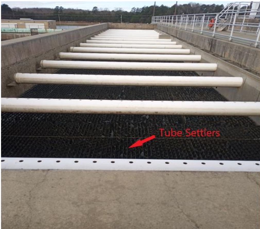
Tube Settlers in the Super Pulsator at the Ward WTP
