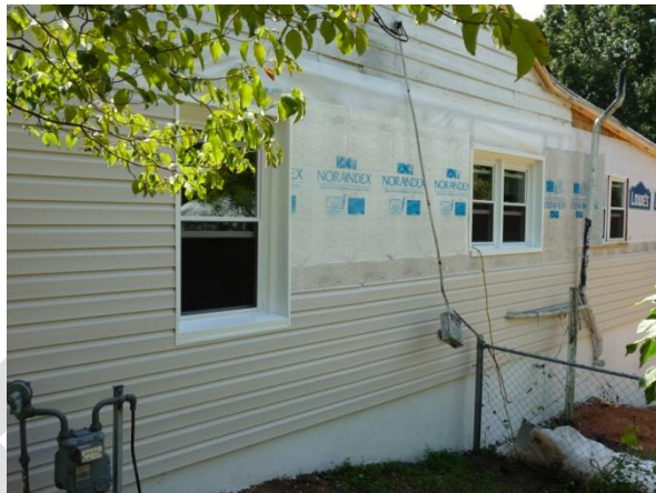
...remediation in process.
