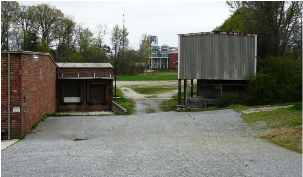
Looking south toward Lincoln Drive. The elevated building and gravel drive are located just south of the public right-of-way.
