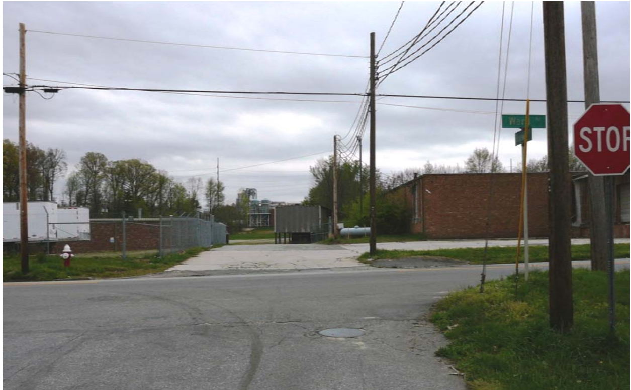
In Rideway Place looking south across W. Ward Avenue to privately improved r/w.
