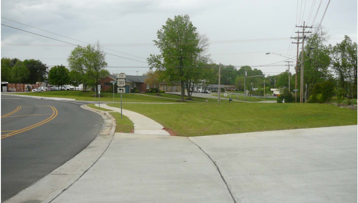
Looking west along the northern limits of Old Winston Road
