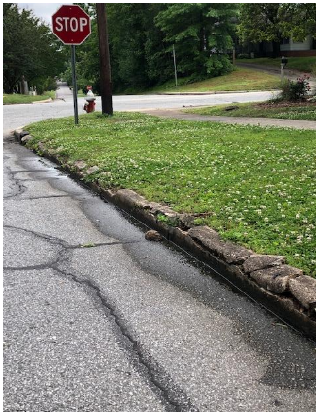
Typical condition of concrete curb requiring removal and replacement
