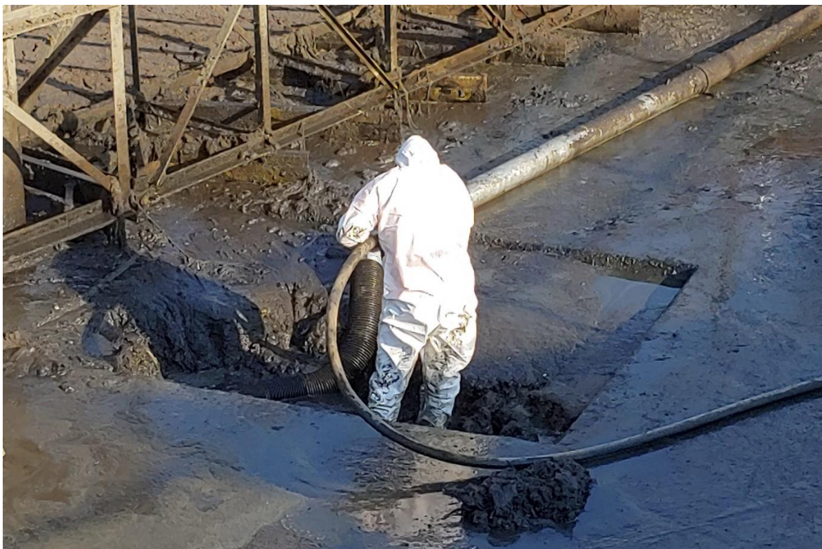
A&D Environmental cleaning out one of the four clarifiers.
