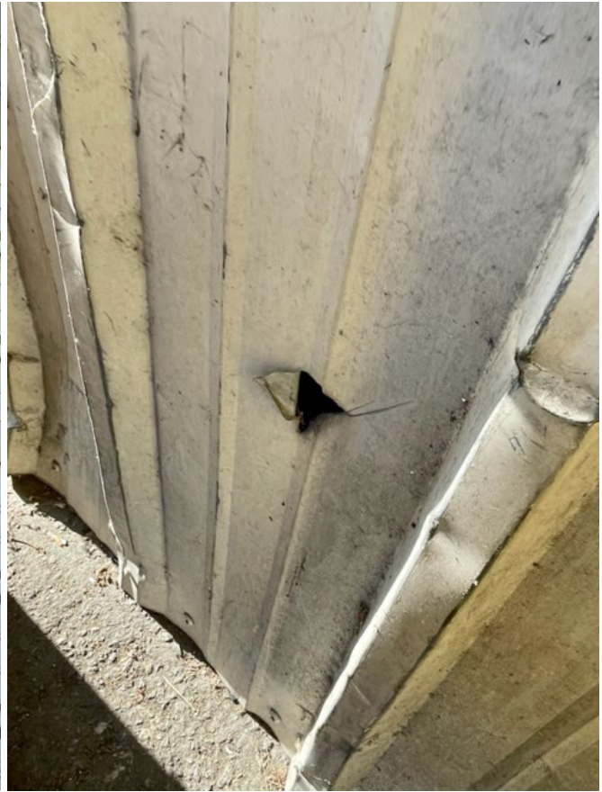
Pictures of damaged exterior siding
