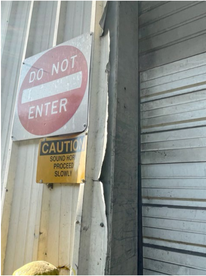
Pictures of damaged exterior siding
