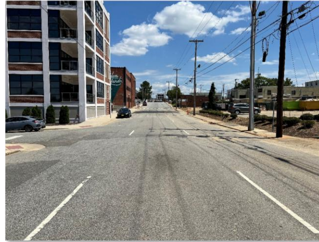
Existing English Road Condition by Congdon Yards
