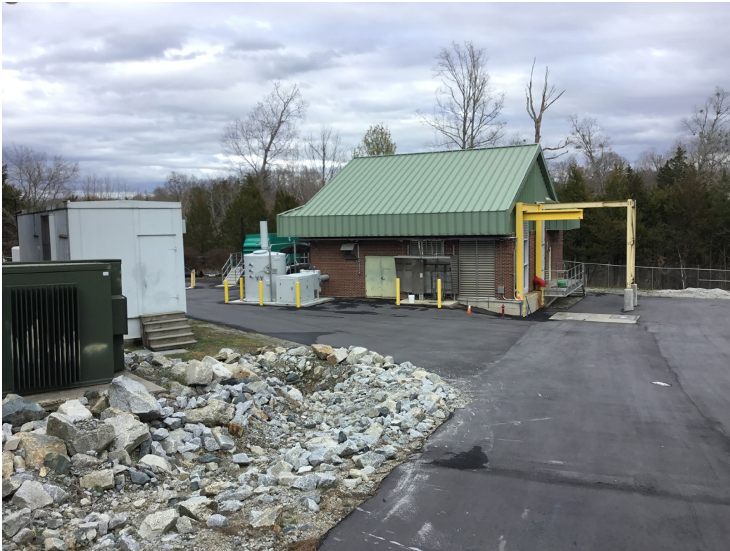
Picture of the Riverdale Pump Station
