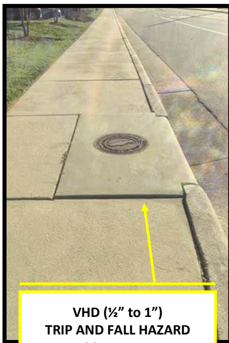
VHD (½" to 1") TRIP AND FALL HAZARD Repairable using Precision Concrete Cutting Process
