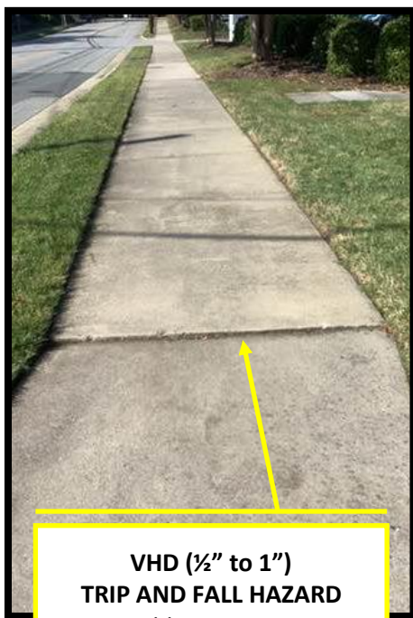
VHD (½" to 1") TRIP AND FALL HAZARD Repairable using Precision Concrete Cutting Process
