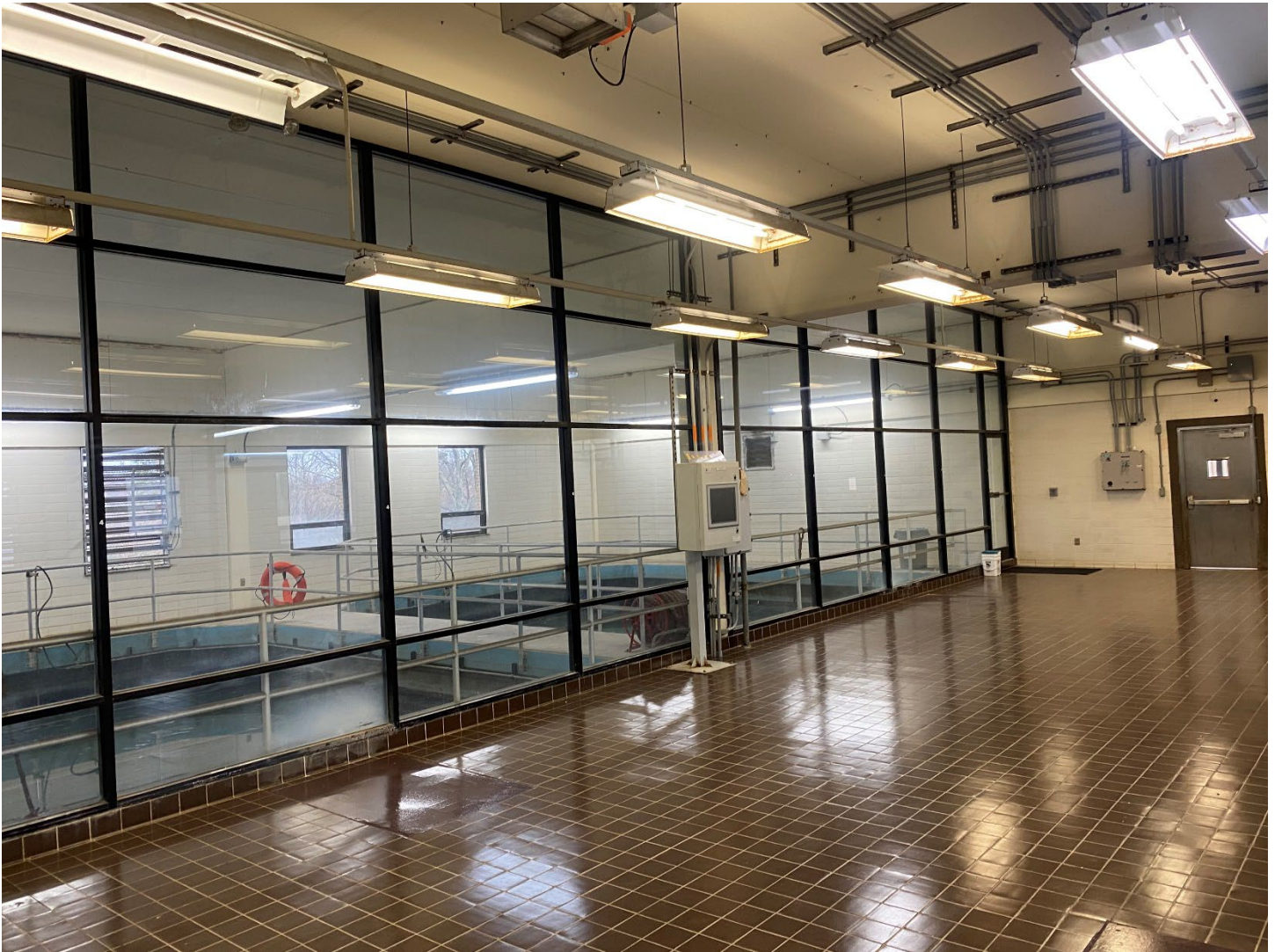
Ward WTP Filter Room
