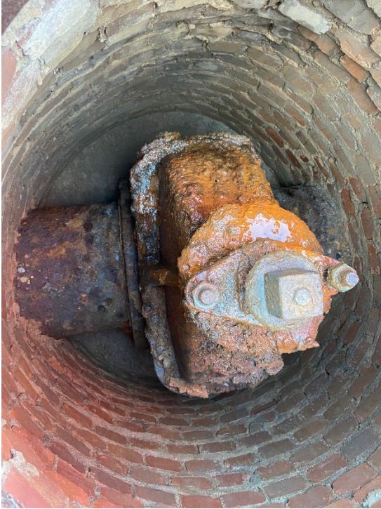
Example of broken water valves
