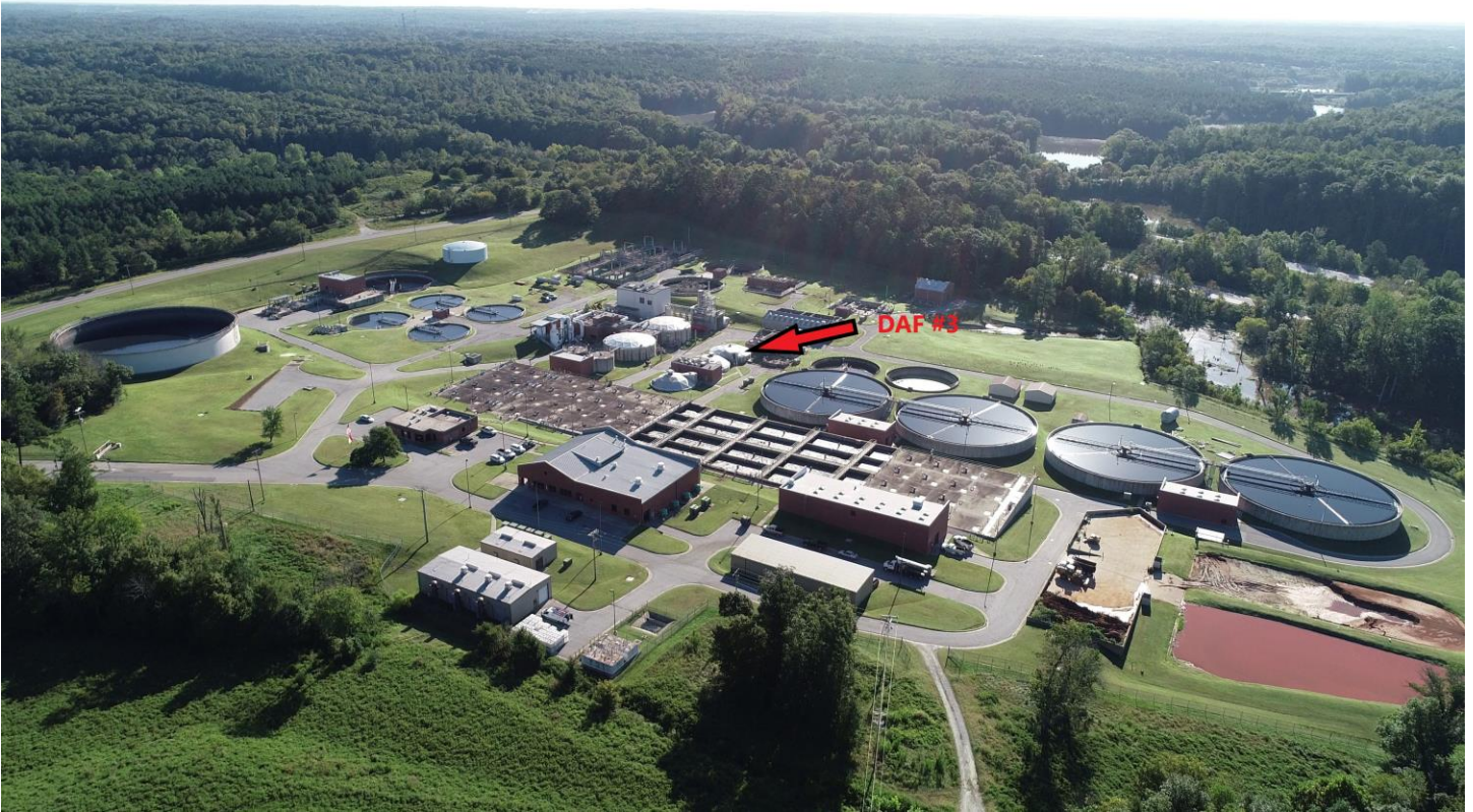
Location of DAF #3 at the Eastside WWTP
