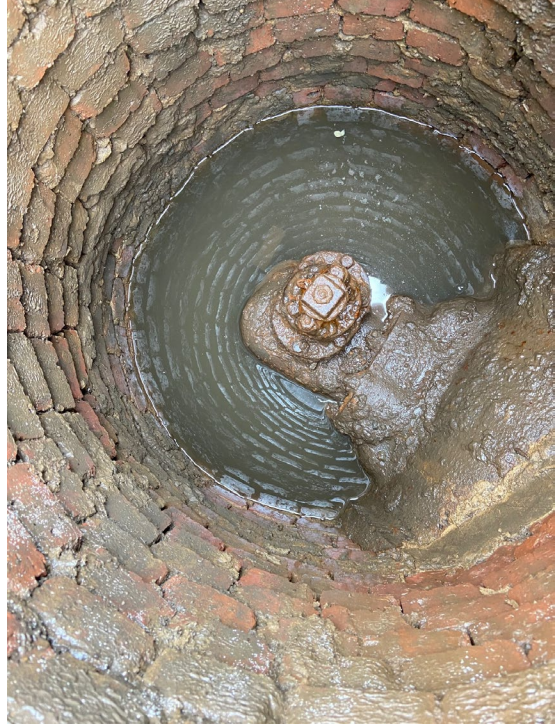
Example of broken water valves
