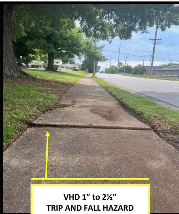
VHD 1" to 2½" TRIP AND FALL HAZARD Repairable using Precision Concrete Cutting Process
