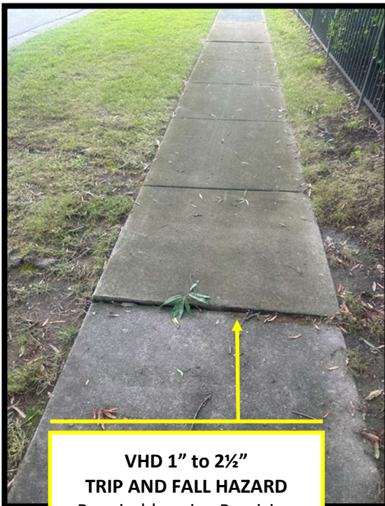
VHD 1" to 2½" TRIP AND FALL HAZARD Repairable using Precision Concrete Cutting Process
