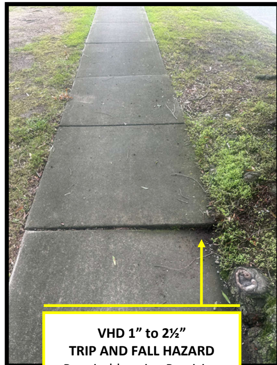
VHD 1" to 2½" TRIP AND FALL HAZARD Repairable using Precision Concrete Cutting Process
