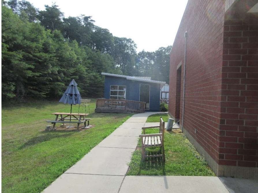
Location of Future Classrooms in Phase 1 to North Side of Main Building
