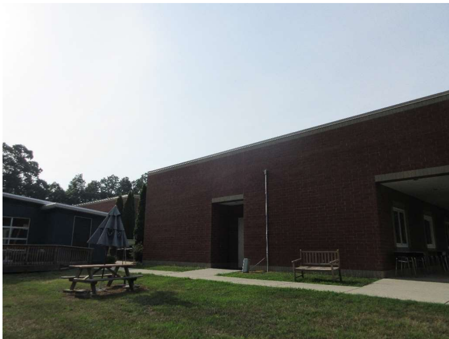
Rear (North) Exterior View of Subject's Current Building
