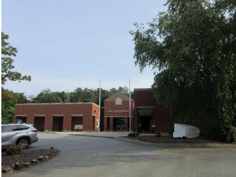
Front (South) Exterior View of Subject's Current Building
