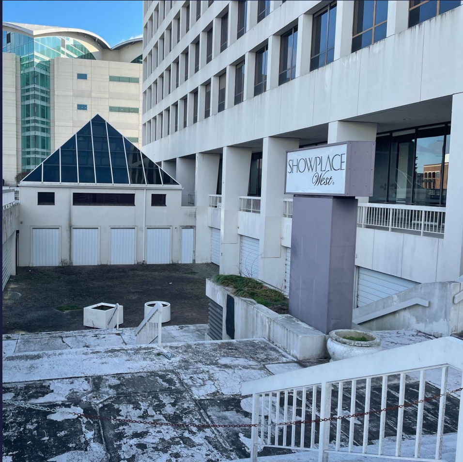
Concrete planters, metal handrails, and sign base
