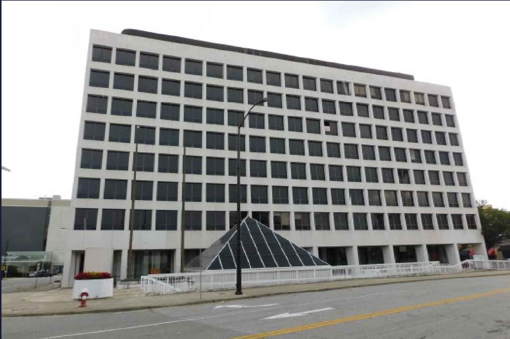
E. High Ave Facade
