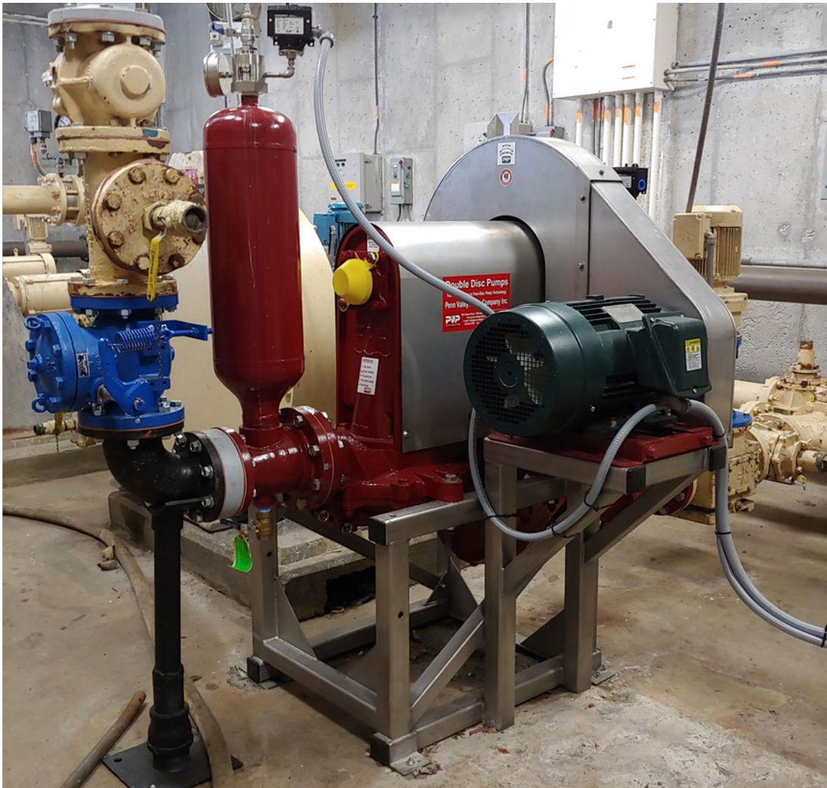
6" Penn Valley Double Disc Pump that has been installed in the Primary Clarifier Building
