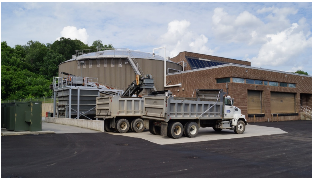
Westside WWT solids building and loading area for dewatered sludge.
