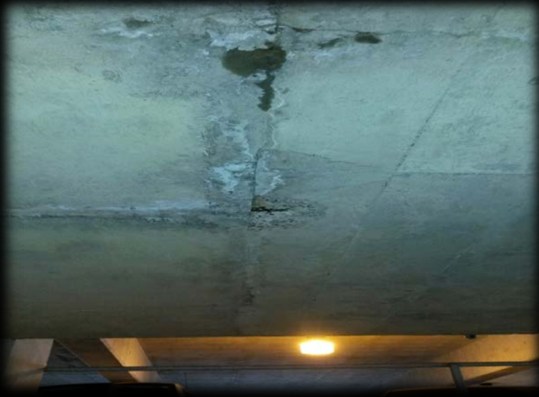
➤ Spalling concrete ceiling (above) and exposed pre-tensioned cable (below)
