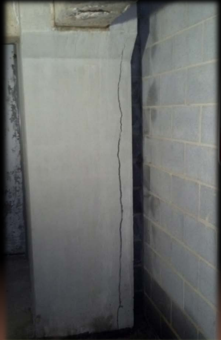
➤ Cracked support column on lower level of Plaza
