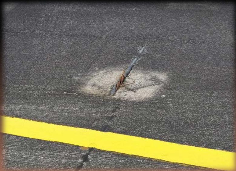
➤ Spalling concrete ceiling (above) and exposed pre-tensioned cable (below)
