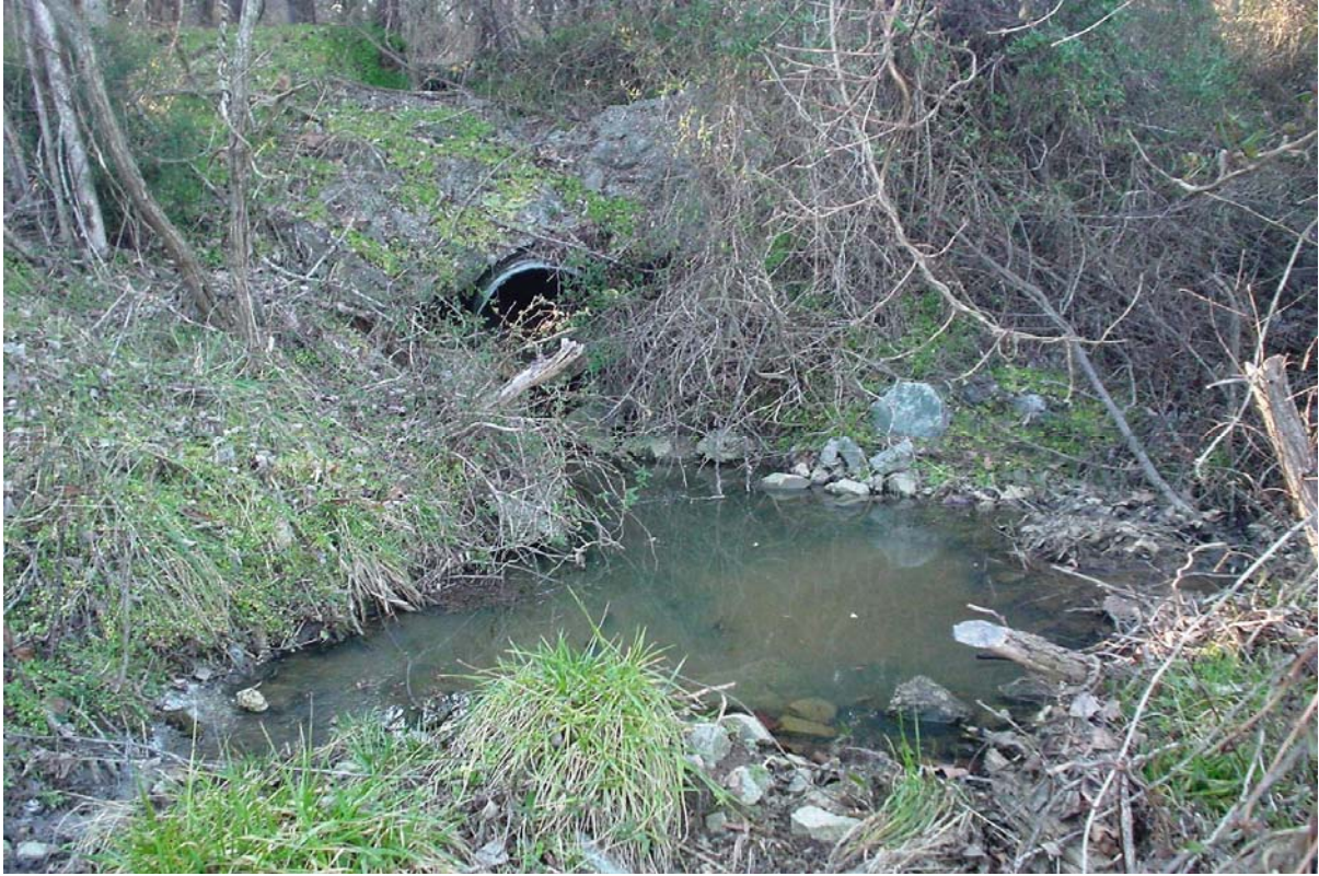
Photo #3 – Pump Station Stream (PSS) where the rerouted NIS will discharge. The pipe shown in the picture will be removed.
