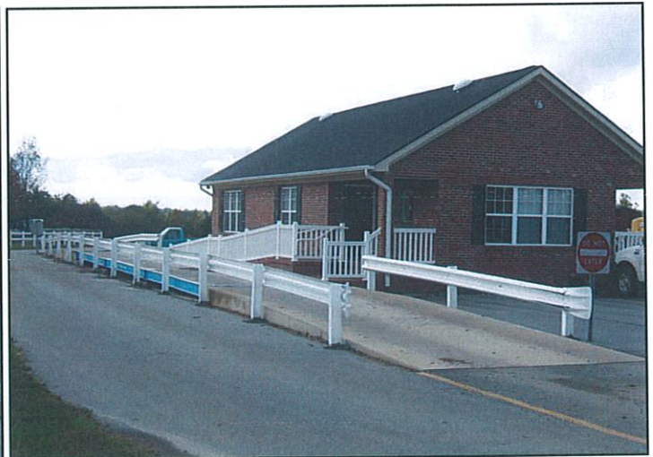
#2 Scale at Ingleside Compost Facility w/ Concrete Deck, Scale, Pad and Ramps
