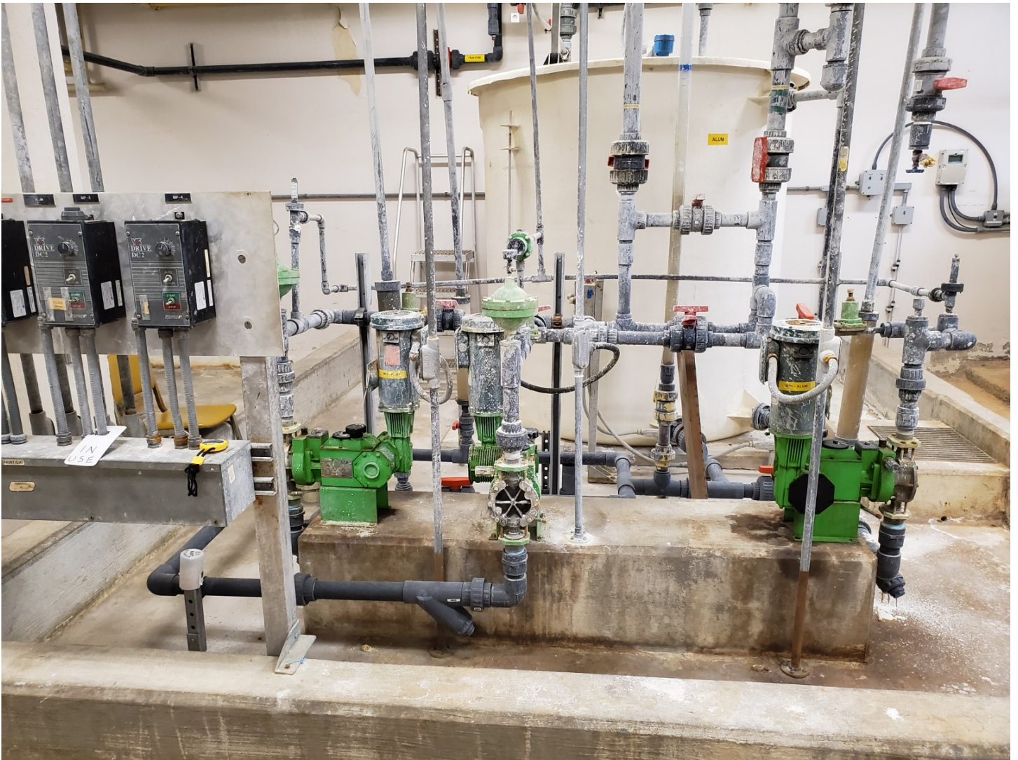
Picture of Existing Alum Feed System
