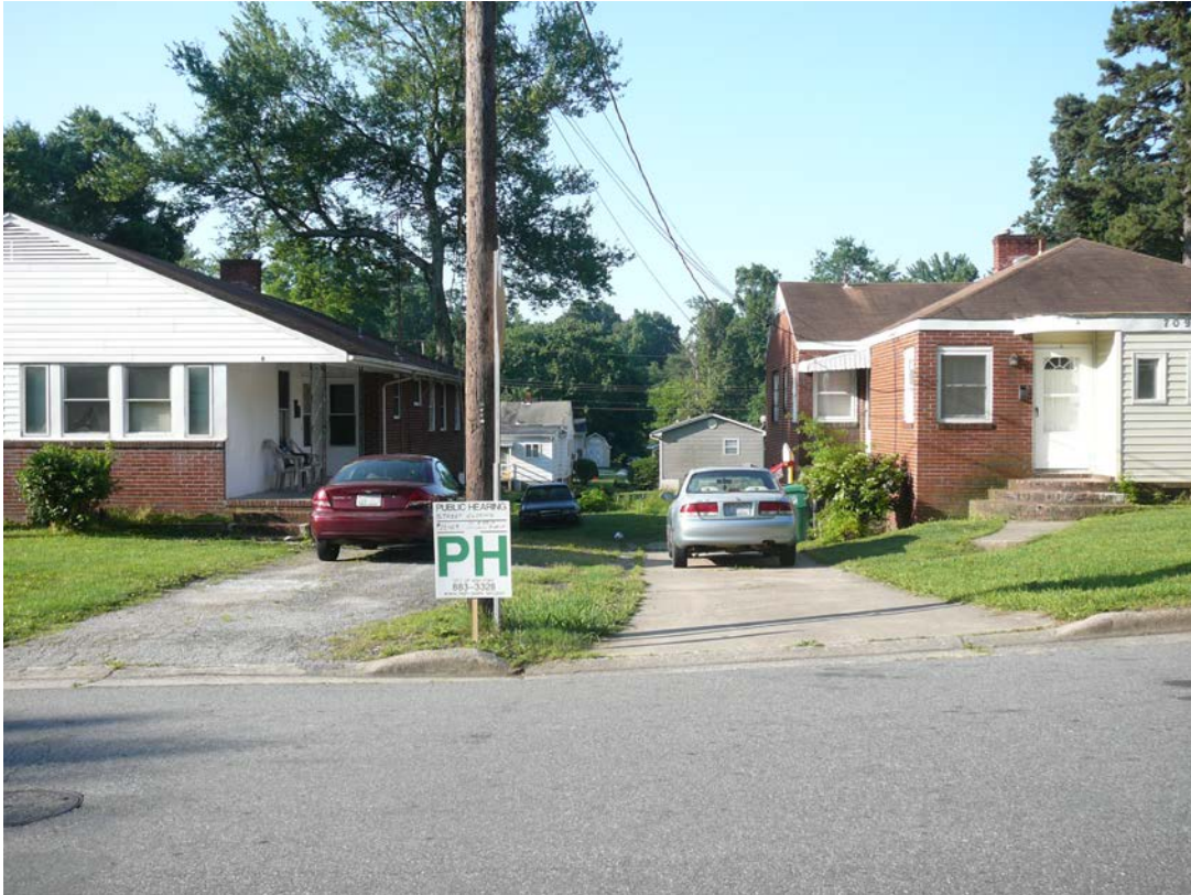
Part B look south from Chandler Avenue
