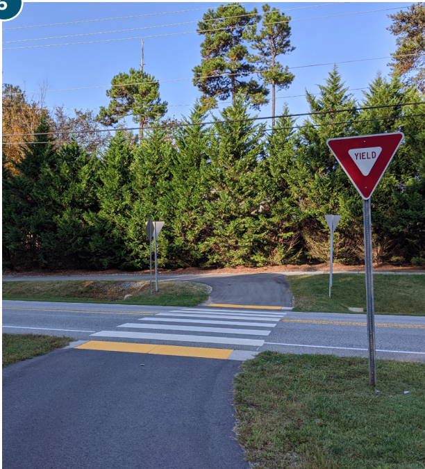
The newest segment of the High Point Greenway begins with an enhanced crossing of Penny Road.
