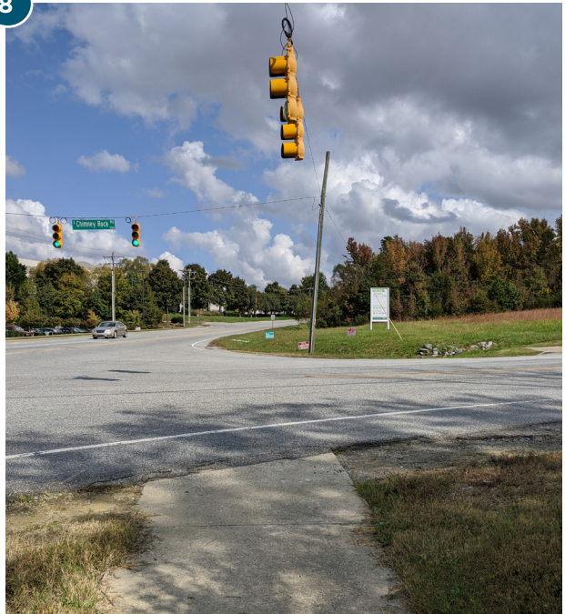
A pedestrian crossing is needed at the northern terminus of the Bicentennial Greenway in High Point, along with branding and wayfinding signage.
