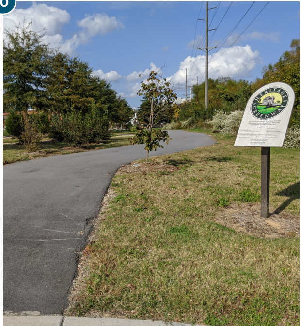
The existing segment of the Southwest Heritage Greenway is in good condition.
