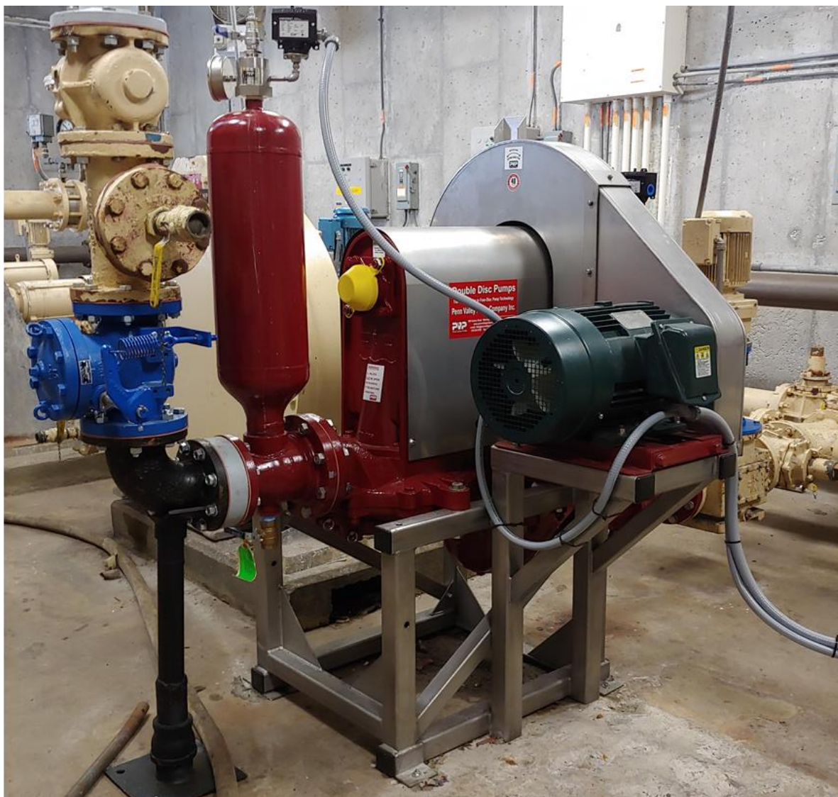
6" Penn Valley Double Disc Pump that was recently installed in the Primary Clarifier Building
