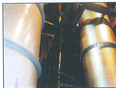
French Broad WRF Incinerator Building
