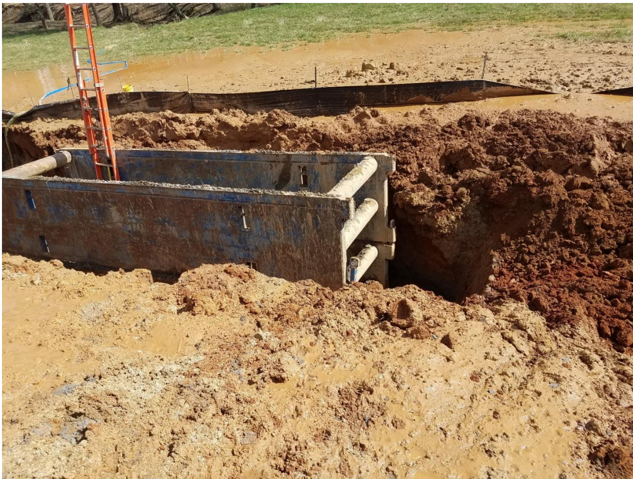
Example of surface water within the project area.
