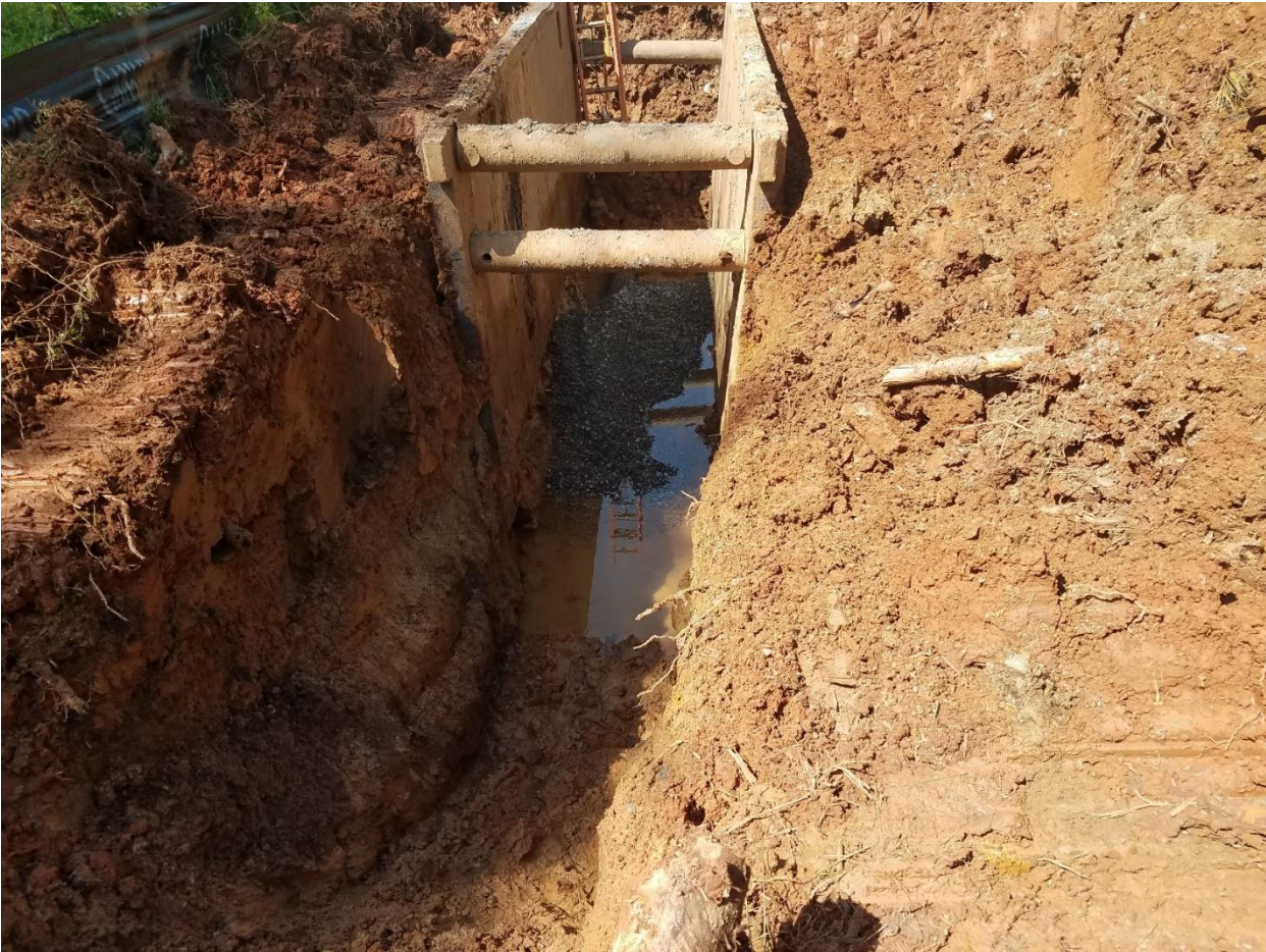
Example of groundwater within the trench.
