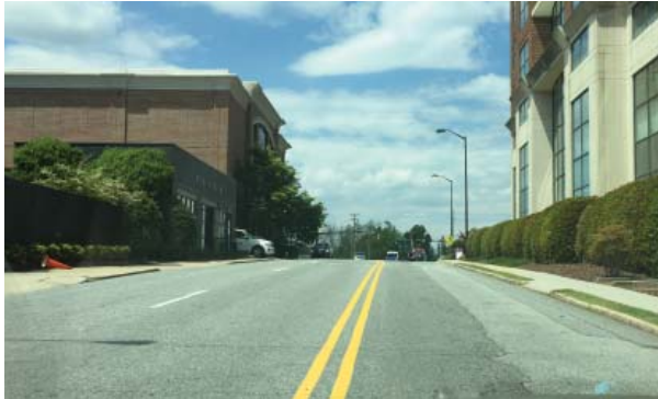
Lindsay Street Upgrade
