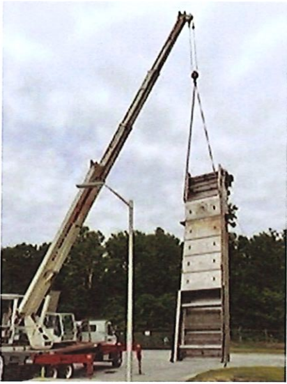
The existing mechanical coarse bar screen at the Westside WWTP being removed for maintenance.
