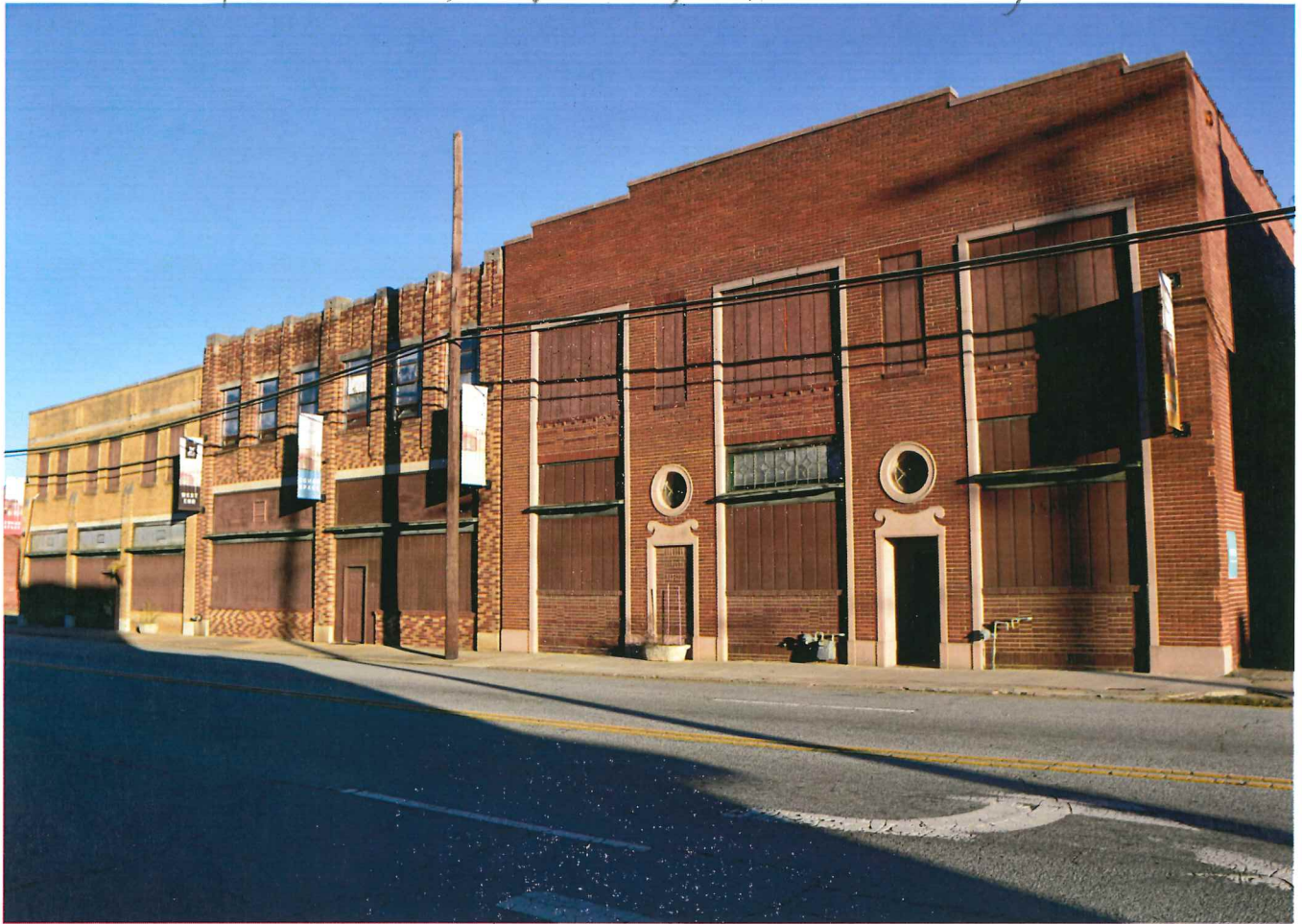
Melrose Hosiery Mill No. 1, High Point, Guilford County
