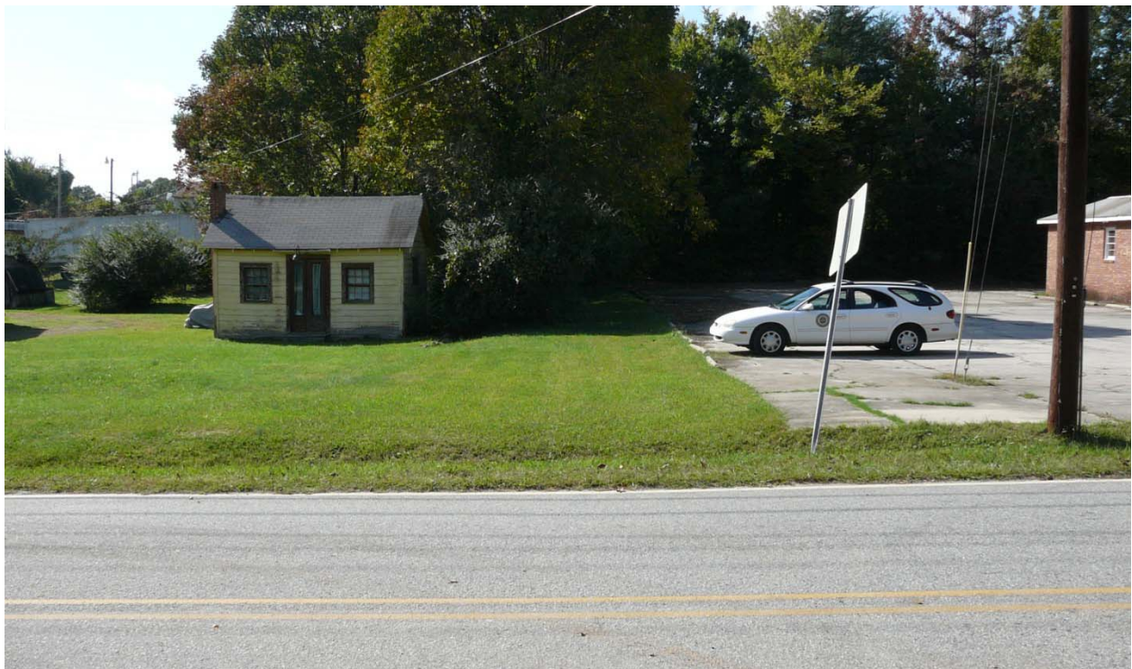
Looking west from New Street. Lawn area and possibly a portion of the Miracle Temple Holiness Church parking lot is within the unimproved right-of-way.
