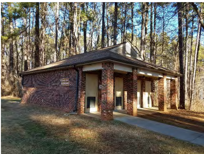
CAMP ANN RESTROOM
