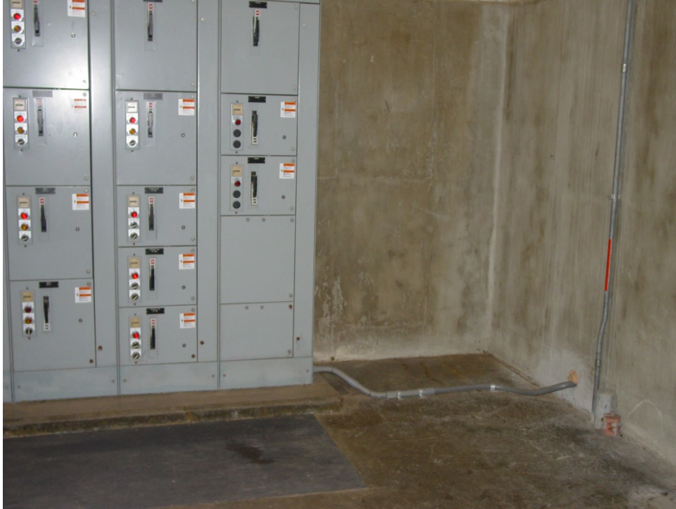
Pictures of temporary repairs out of Master Control Center (MCC)
