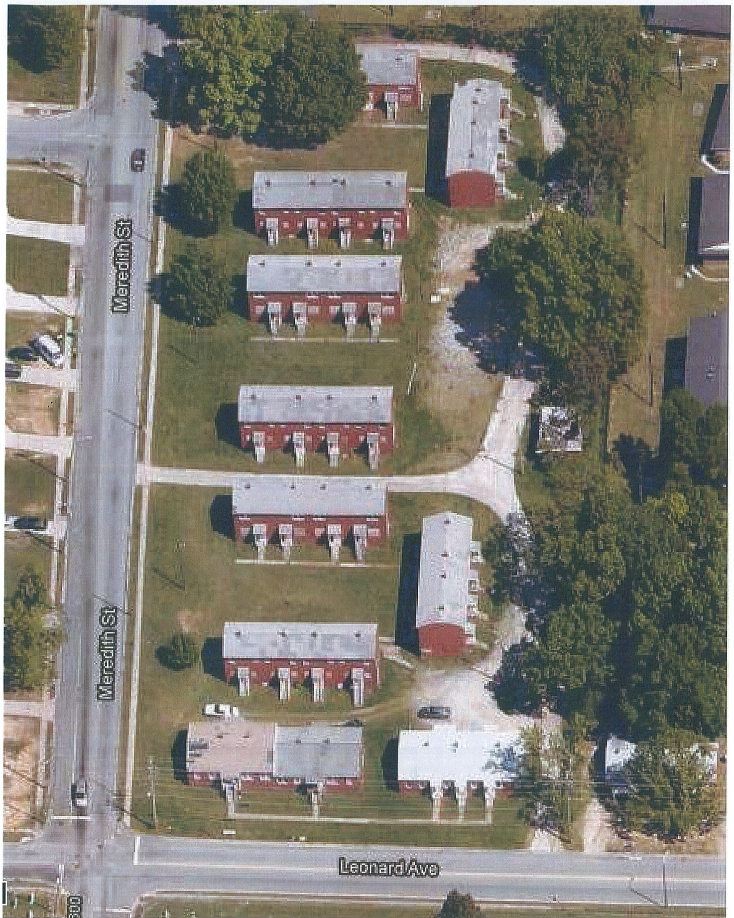
515 Meredith St., Apartments High Point, NC (39 units)
