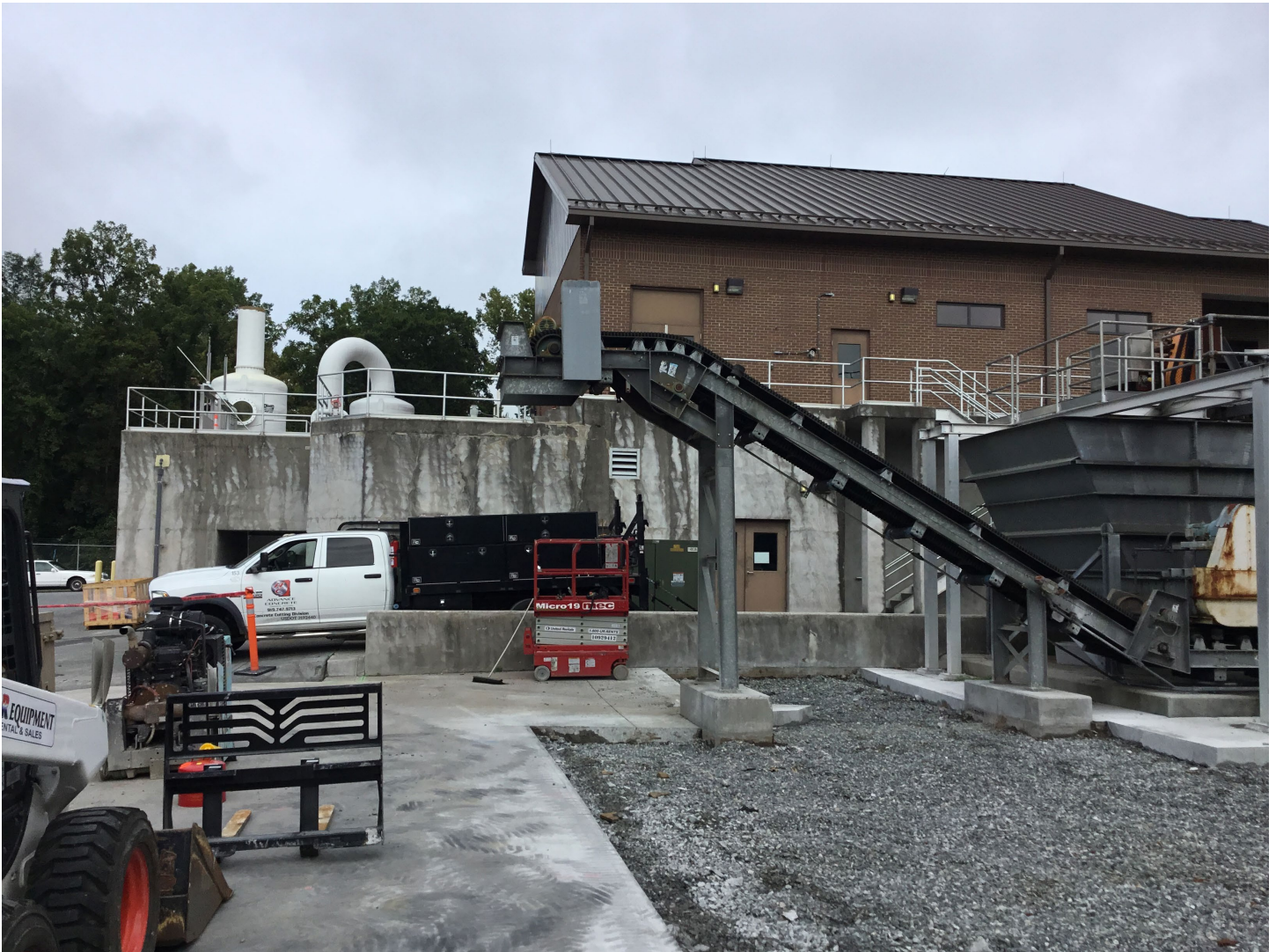
Truck loading area prior to new concrete pour
