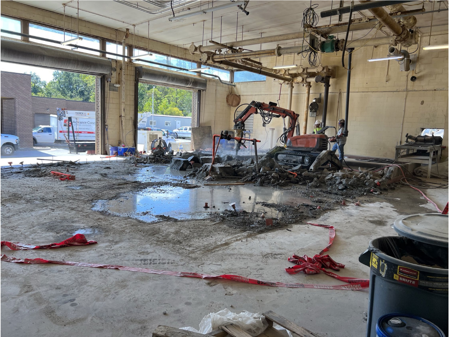
Demolished centrifuge platform and concrete pad
