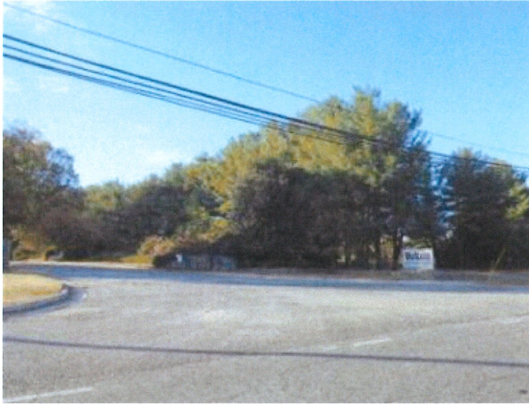
View of Thompson Arthur Asphalt plant located at 2859 Highway 66 South, Kernersville, NC 27284
