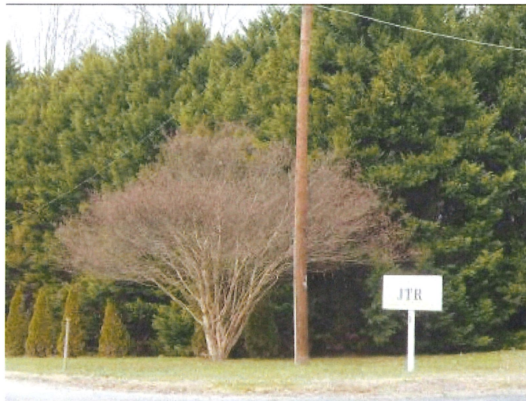
Additional view of Entrance to JT Russell Asphalt Plant Conover, NC
