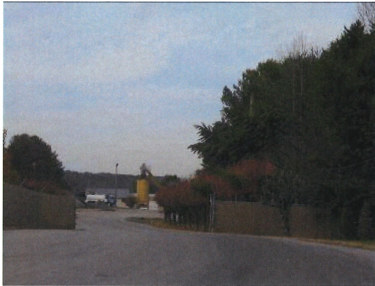
JT Russell Asphalt Plant located at 201 Herman Sipe Road, Conover, NC
