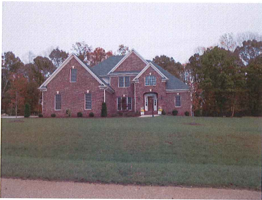
Front View of 7022 Carriage Cove Drive, Oak Ridge, NC (Guilford County)
