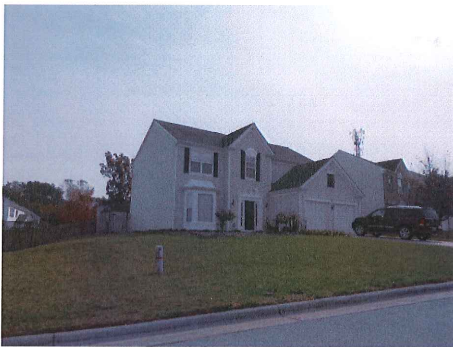
Photo of Lattice Style Cell Tower at 4401 Johnson Street High Point, NC
