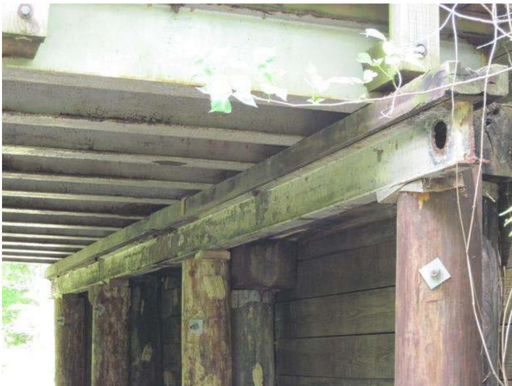
Crutch bent at end bent 2.
