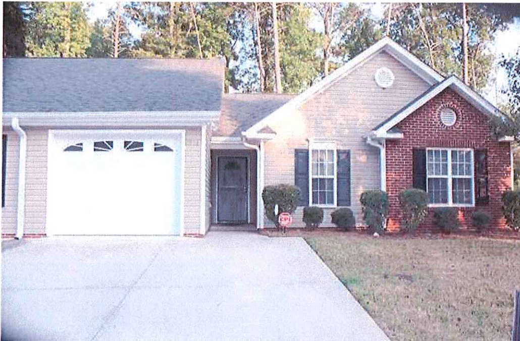
Front View of 7871 Woodpark Drive, High Point, NC
