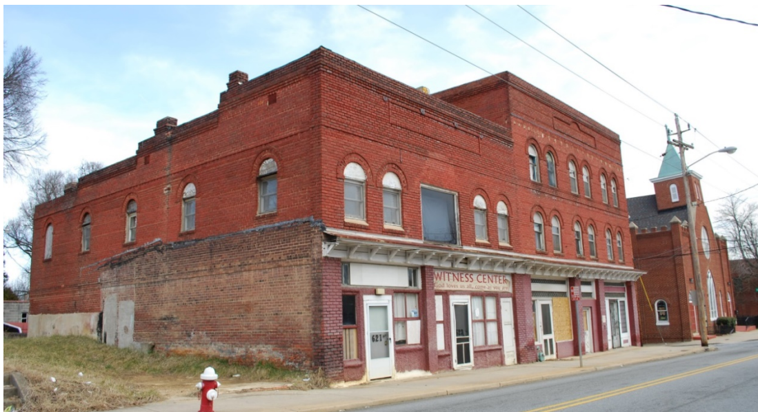
Kilby Building (in foreground)
