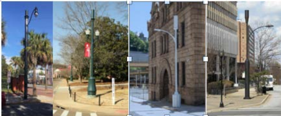
FIGURE 4.3.3.F2 CONCEALED SMALL WIRELESS FACILITIES
