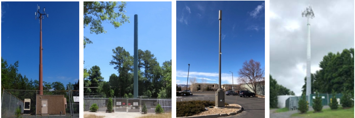
FIGURE 4.3.3.F1 STEALTH WIRELESS TELECOMMUNICATIONS FACILITIES PAINTED WIRELESS FACILITIES
