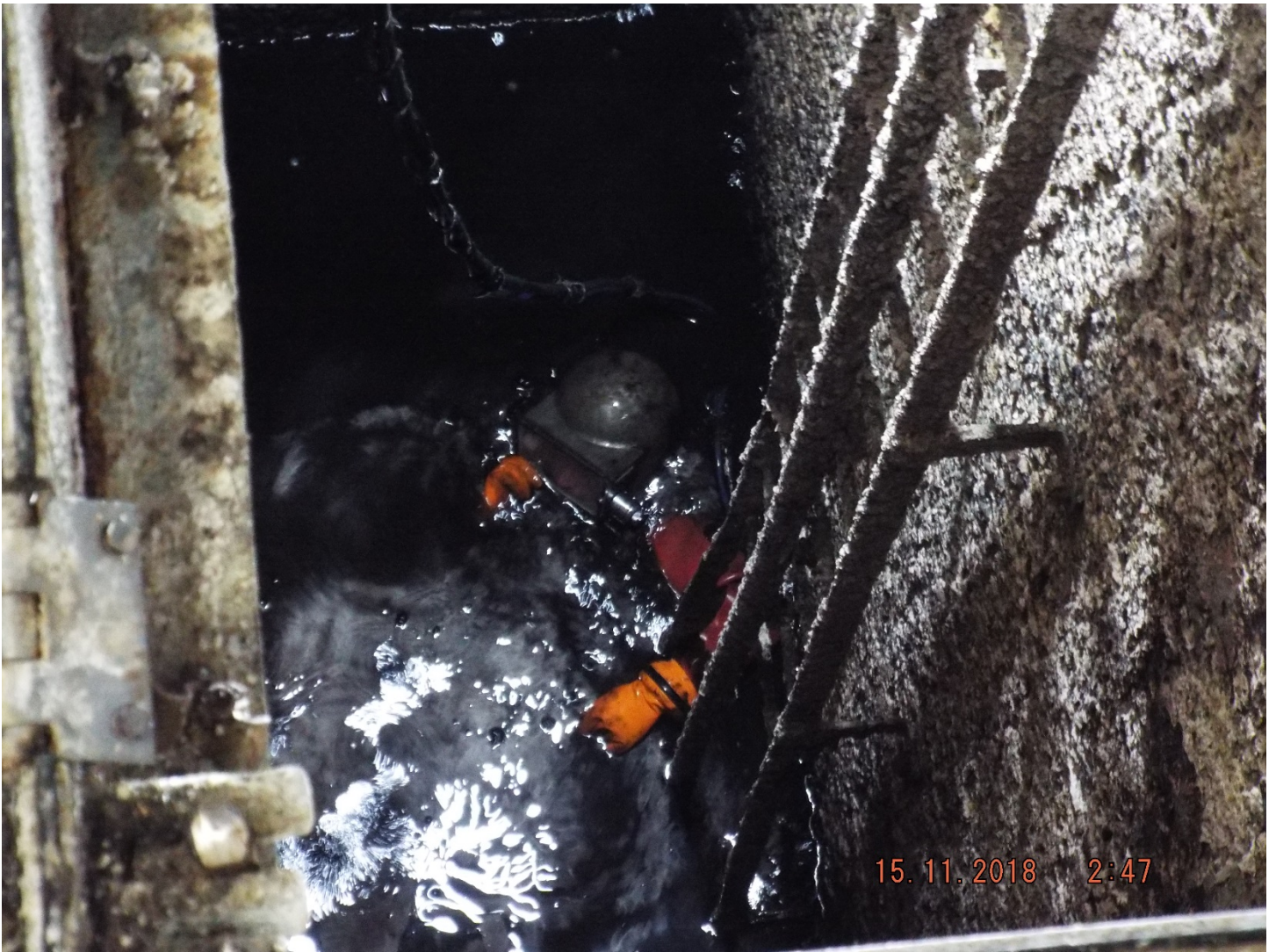
Diver in Wet Well
