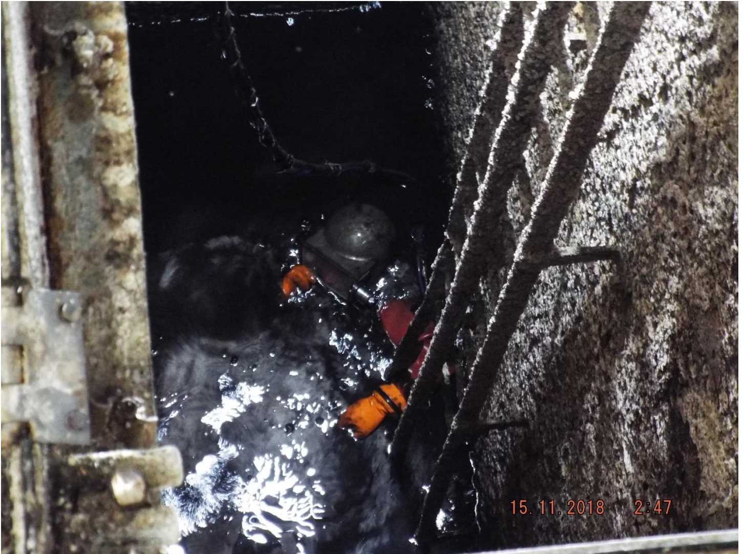
Diver in Wet Well
