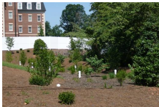
Biocell stormwater control device on Guyer Street
