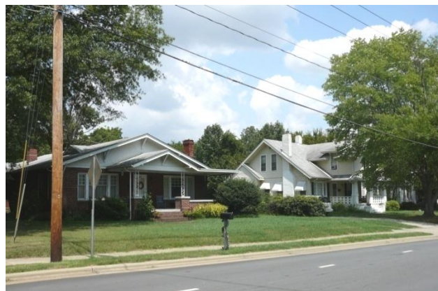
Example of houses on the north side of Montlieu Ave. that are recommended for reuse by the university
